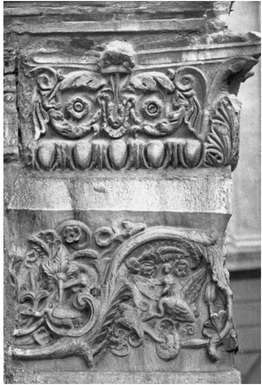
Figure 125 Panagia Gorgoepokoos. Roman anta capital and part of a frieze, in secondary use, at the southwest corner of the church.
